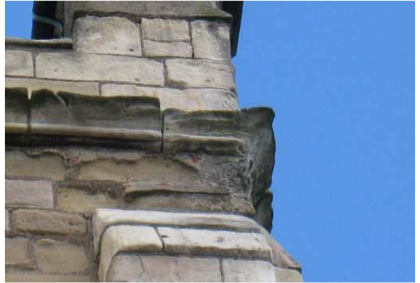
ERODED CORNICE
