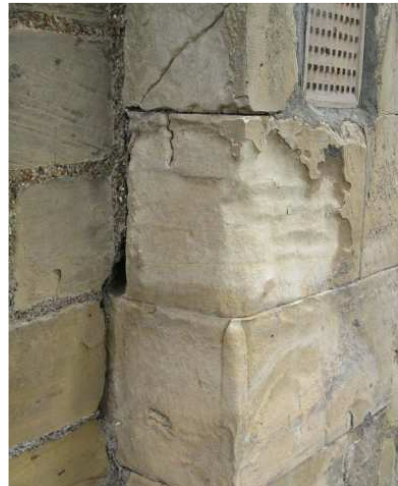
BUTTRESS EROSION
