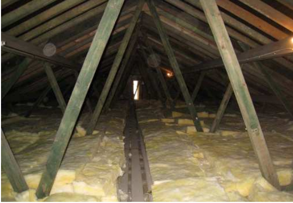
NAVE ROOF SPACE
