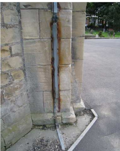
EXPOSED CONDUCTOR
