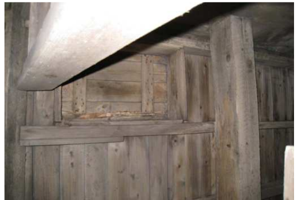
TOWER ROOF CONSTRUCTION
