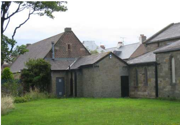
HALL, BOILER HOUSE & LINK
