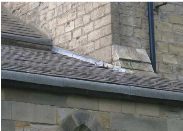
ORGAN LOFT ABUTMENT TO EAST NAVE GABLE
