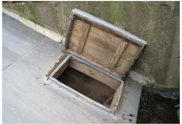
TOWER ROOF HATCH
