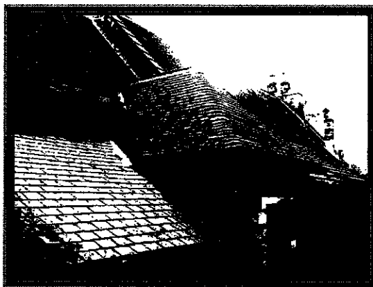
(Missing lead flashing to North elevation)
