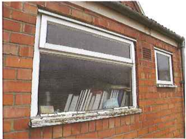
10. North wall, external view (window detail)
