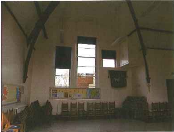
5. Internal view looking South
