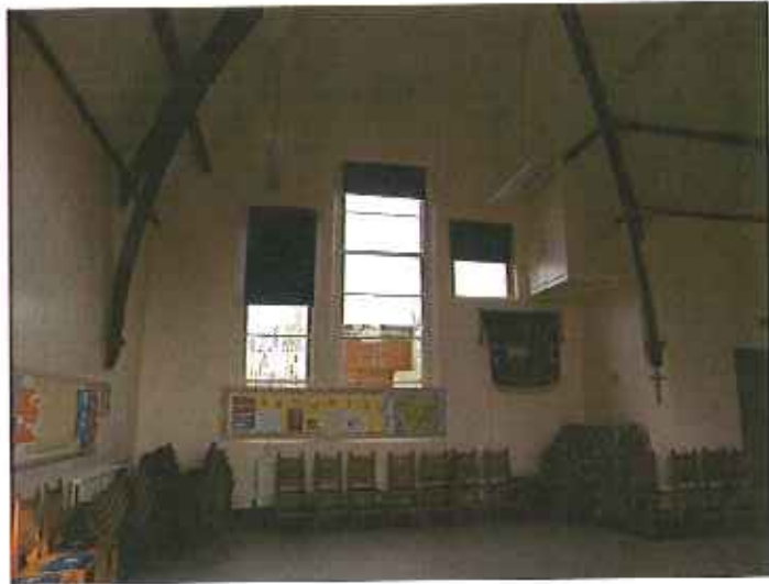
1. Internal view looking North
