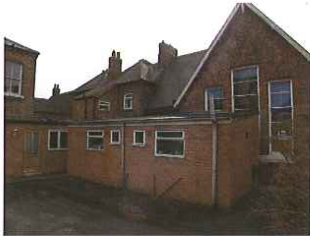
13. General external view of North wall and outbuildings
