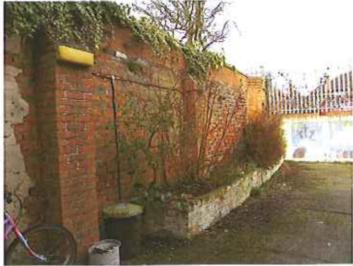
3. West boundary wall, yard area to North of church
