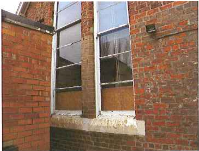
6. External view, North wall of church
