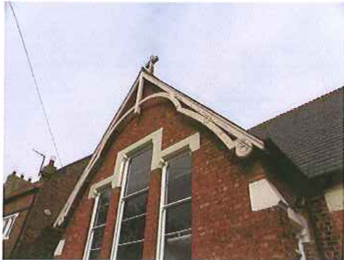
15. South facing gable (detail)
